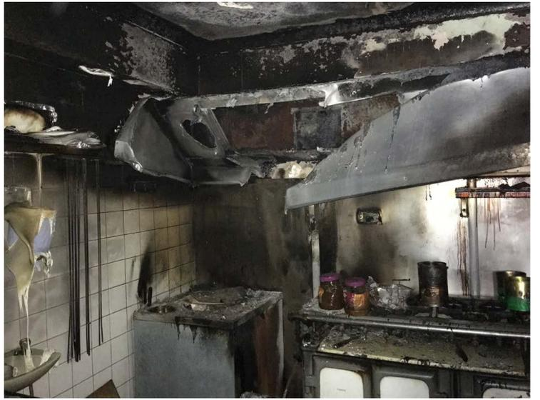
Non-fire resistant ductwork systems can be responsible for allowing the initial spread of fire and smoke between compartments. The correct use of fire-rated ductwork will maintain fire compartmentation and assist in the safe dispersal of hazardous smoke and fumes.
