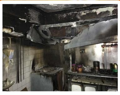
Non-fire resistant ductwork systems can be responsible for allowing the initial spread of fire and smoke between compartments. The correct use of fire-rated ductwork will maintain fire compartmentation and assist in the safe dispersal of hazardous smoke and fumes.
